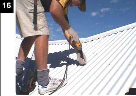
Remove any Roof Sheeting Tek Screws from the area around where the Sky Tunnel is going to be installed.
