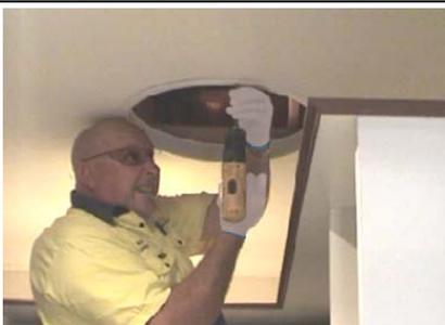
Insert the Ceiling Frame and attach with the 50mm Supachip Screws and plastic lugs provided. The plastic lugs are placed on the top side of the ceiling. Fasten the screws through the holes in the ceiling frame, the ceiling and into the white plastic lugs tighten.
