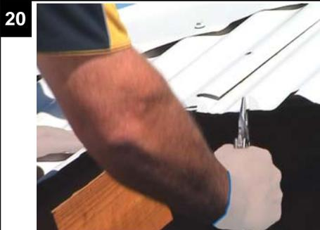
Bend both sides of the cut downwards, to create an overlap, which closes off the corrugations on the high side.
