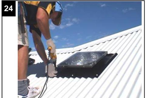
Re-install any Roof Sheeting Tek Screws that were removed.
