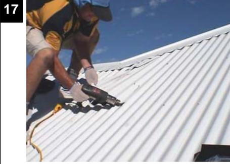
Cut out along the lines that were marked, ensuring cuts finish on the highest point of a corrugation.
