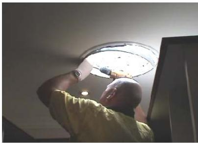
Fit the White Plastic Flexi-tube Locking Ring into position with the Countersunk Screws provided.
