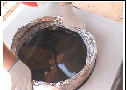
Push the Stainless Steel Ring (with the Flexi-tube fitted) into the underneath of the Black Breather Frame, lining up the slots in the Ring with the Lugs in the Breather Frame.
