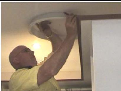
Using the up-stand of the Ceiling Frame as a template, or using the template on your Ceiling Parts Box, mark the hole size on the ceiling with a pencil, ensuring the nail hole is at the centre.
