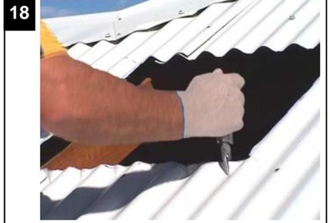
On the low side of the hole, bend up all of the lowest points on the corrugations to prevent any water blowing back up the corrugations, and under the Soaker Tray into the roof space.
