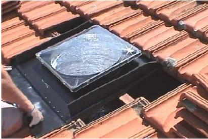
Ensure the rear portion of the Soaker Tray is underneath the tiles behind and the front portion is on top of the tiles.
