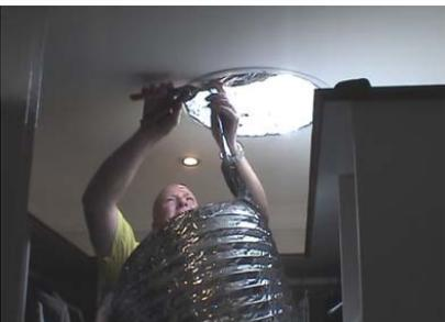
Reach through the Ceiling Frame and pull the Flexi-tube through the Ceiling Frame and into the room. Continue pulling until it is tight, the wires will lock onto the lip at the top of the Ceiling Frame.
