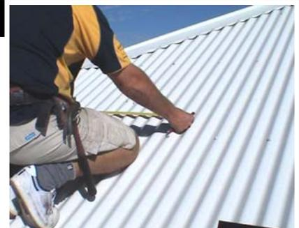
For each Sky Tunnel, double check all your measurements on the roof and the Soaker Tray to ensure you will get full coverage over the hole, with plenty of overlap on all sides. Back of Soaker Tray will be under the Roof Sheets.
