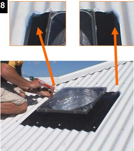
Using a Roof & Gutter Silicone, seal both corners on the high side of the Soaker Tray.
