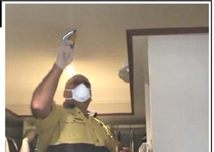
Cut neatly along the pencil line on the ceiling with a keyhole saw. You should wear protective equipment such as Safety Glasses and mask where possible, as dust and debris may fall whilst cutting. Hold the middle of the circle you are cutting when nearing the end to stop the panel falling out.
