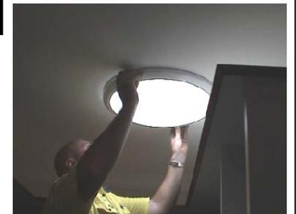
Fit the Diffuser into position. Ensure you line up the Magnets in the Diffuser Holder with the Magnets on the face of the Ceiling Frame.
