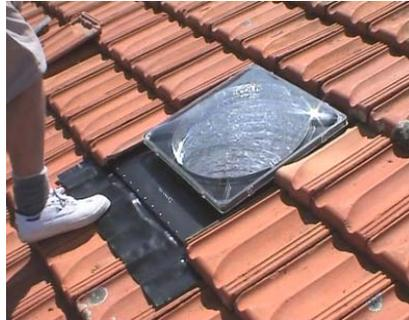
Gently mould the corrugated flashing at the front of the Sky Tunnel to match the profile of the tiles.
