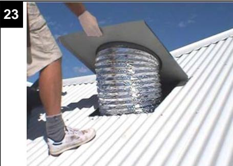
Lower the Sky Tunnel into position. Be careful to make sure the Flexi-tube does not catch on the Roof Sheeting.
